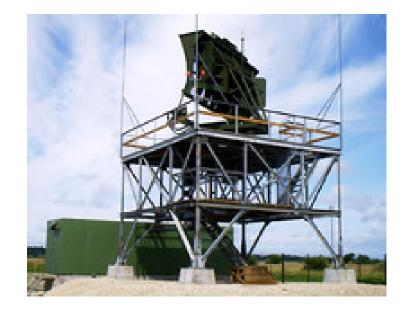
Sensors / EW: - ASR-7 GCA - Radar, Radar, Air Search, 2D Medium-Range, Max range: 111.1 km
